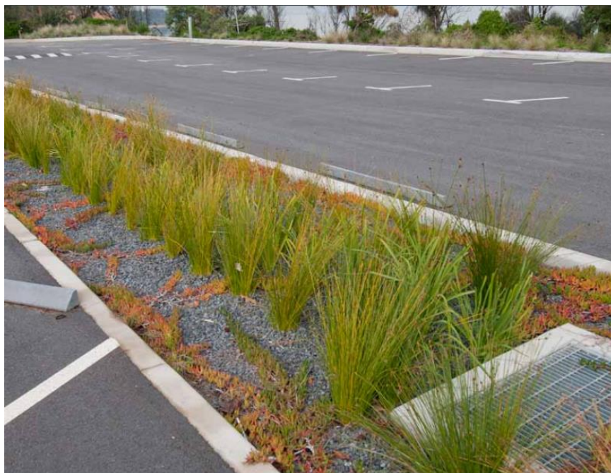
Figure 3.7: Vegetated Swale – Source: CSIRO (2005)
